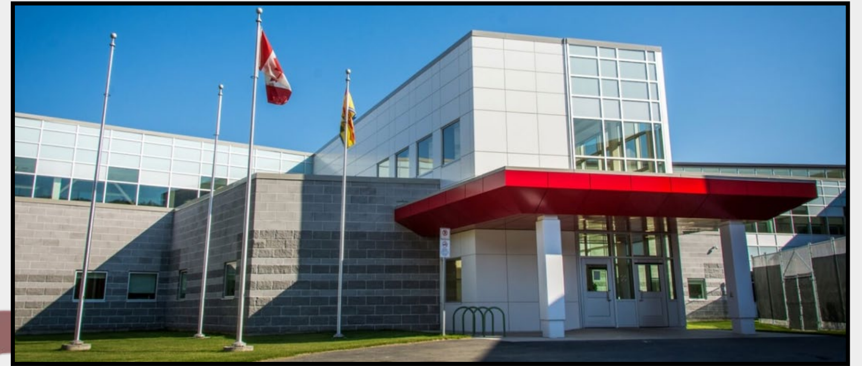
Centre Hospitalier Restigouche Hospital Centre
